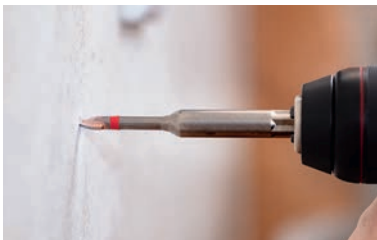
1. Drill hole in porcelain / gres tiles with C PROTECTOR
